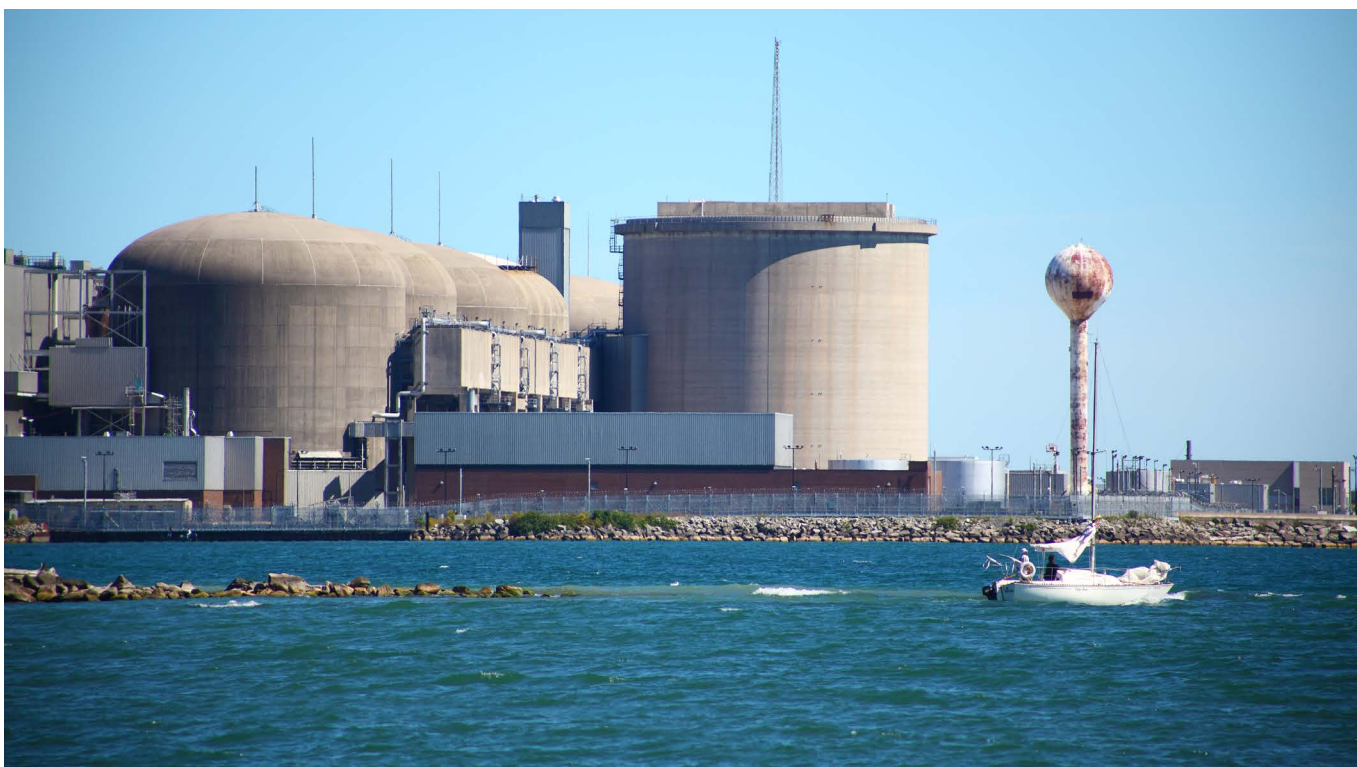
Ontario's Pickering Nuclear Generating Station
