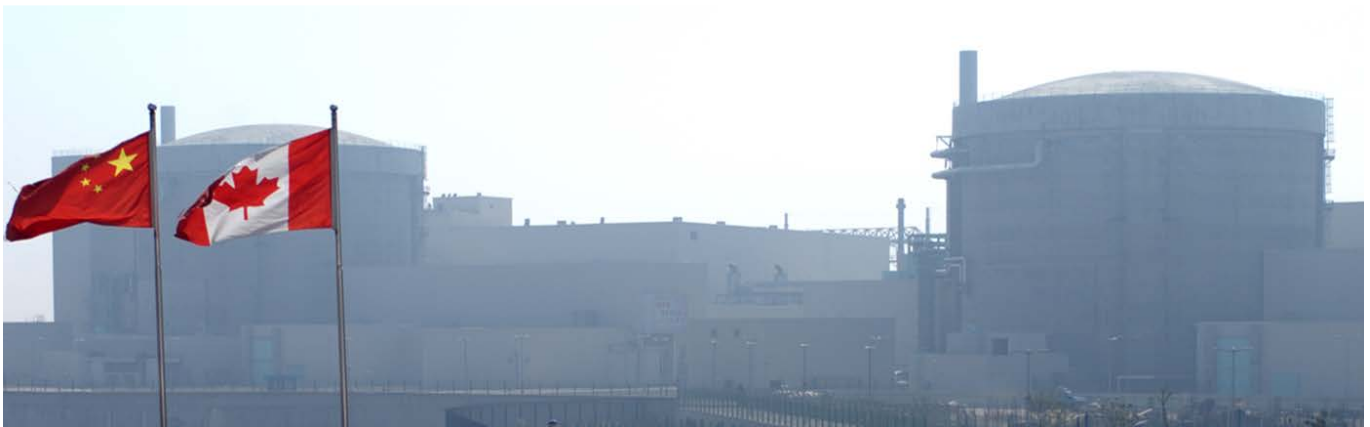
Chinese and Canadian flags at Qinshan Nuclear Power Station, Zhejiang, China
